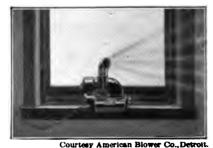
"Sirocco" Fan Blowing into Room.
